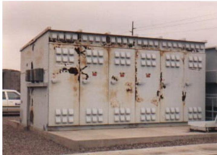
Typical Chloride Induced Coating Failure
